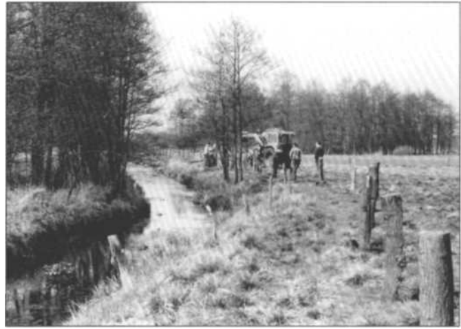
Reconstruction work to improve otter habitat along a channelized stream in West Germany (Photo courtesy of Aktion Fischotterschutz).
