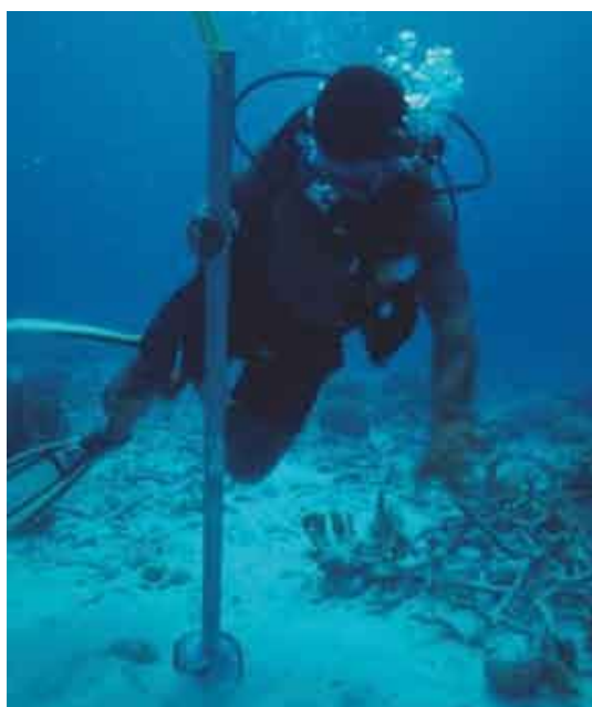
A marine park ranger installs a mooring buoy which will reduce anchor damage to corals in Bonaire Marine Park (Netherlands Antilles). Photo: Dee Scarr
