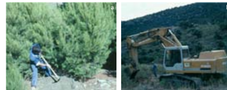
Site preparation : a) manual b) an excavator, Photos by: R. Hierro
