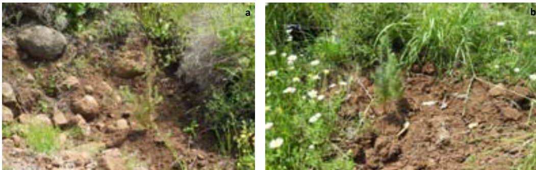
Plantation after site preparation: a) manual b) excavator Photos by: M. Navarrete, IDAF
