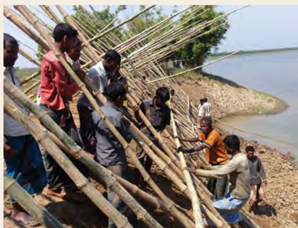
Dam construction by local community
