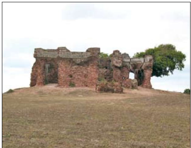
Figure 3.8 – First British Governor Frederic North's circuit bungalow, which was based on Greek Doric architecture. It was later used as a circuit bungalow for government officers. (Sampath Goonatilake © IUCN)
