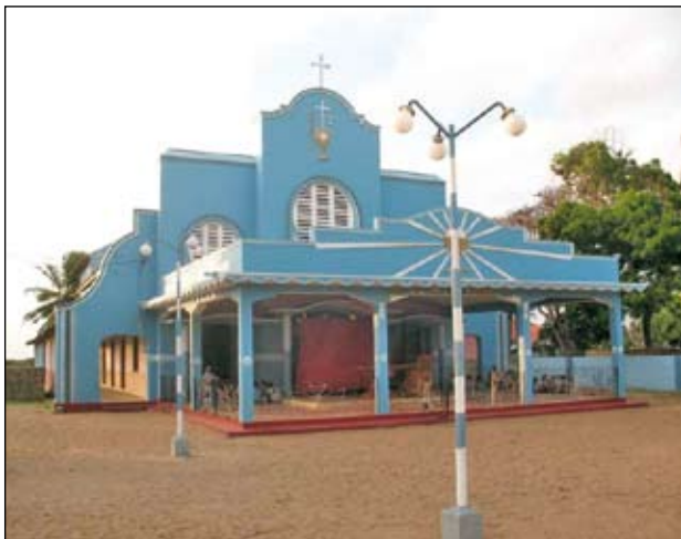
Figure 3.7 – St. Mary's church, Arippu (Sampath Goonatilake © IUCN)
