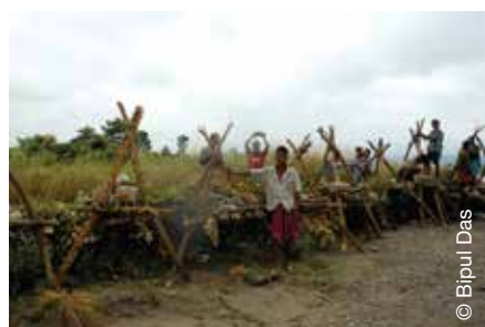
Step 4: Construction of deflectors (called porcupines) using locally available materials and through collective labour.
