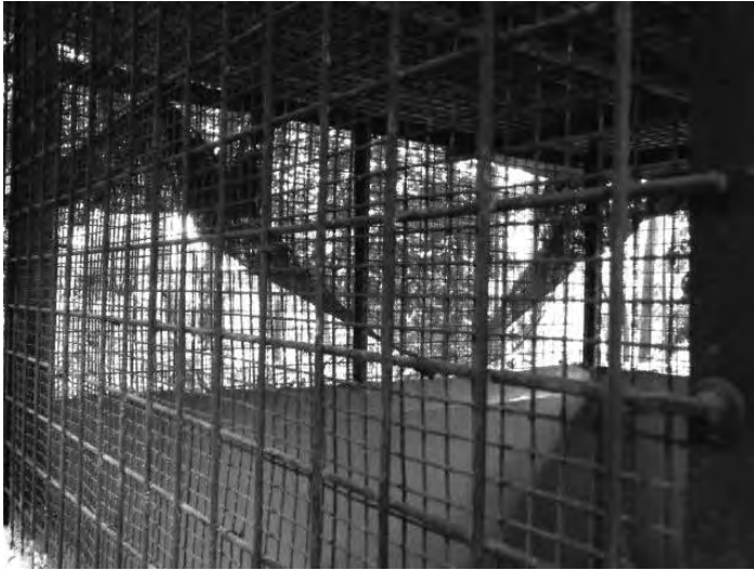
Figure 2: The roof and upper portions of the wall are made of 2 x 2 in galvanised iron mesh, overlaid with 0.5 x 0.5 in stainless steel mesh
