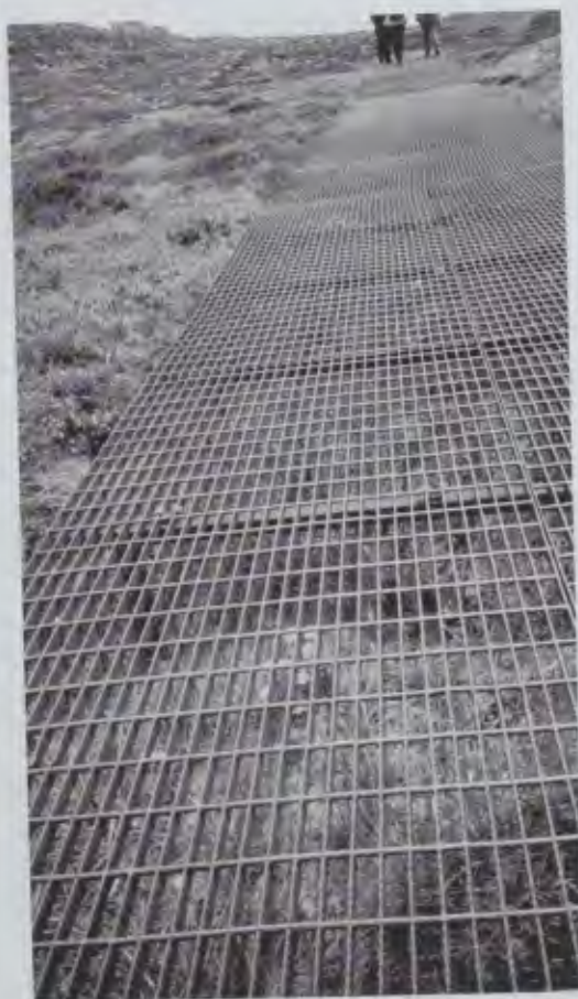
Light-transmitting steel-mesh elevated walkway, alpine area, Kosciuszko National Park, New South Wales, Australia
