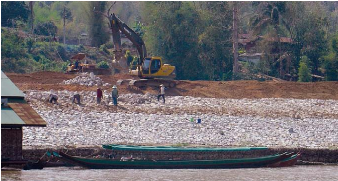
Embankment work in Thailand. © Phaknakhone Rattana/IUCN
