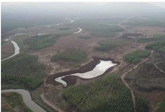
Fig 4. (a) Photo of the area before restoration (© LCRC)
