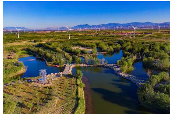
Fig 5. (b) Aerial photo of the riparian area after ecological buffer zone construction (© LCRC)
