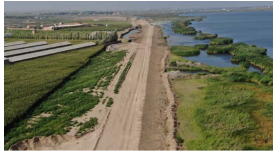
Fig 20. (b) Aerial photo of the riparian area after ecological protection belt management (© LCRC)
