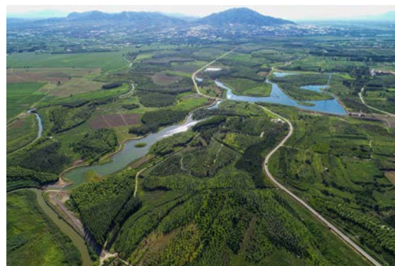
Fig 4. (b) Photo of the area after vegetation restoration and puddles connection engineering (© LCRC)
