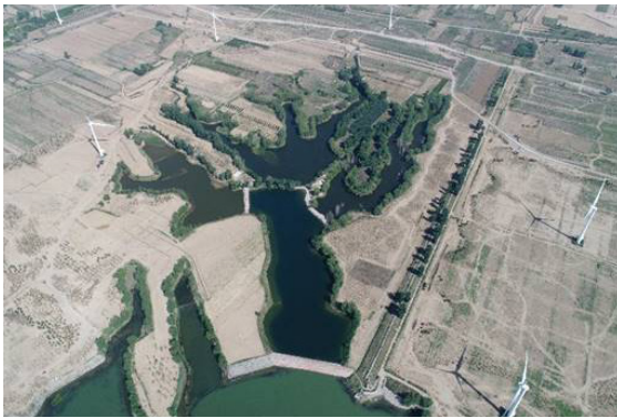
Fig 5. (a) Aerial photo of the riparian area before ecological buffer zone construction (© LCRC)
