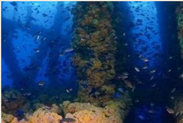
Marine biodiversity colonising offshore facilities of TotalEnergies located in Gabon Bleu marine protected areas
