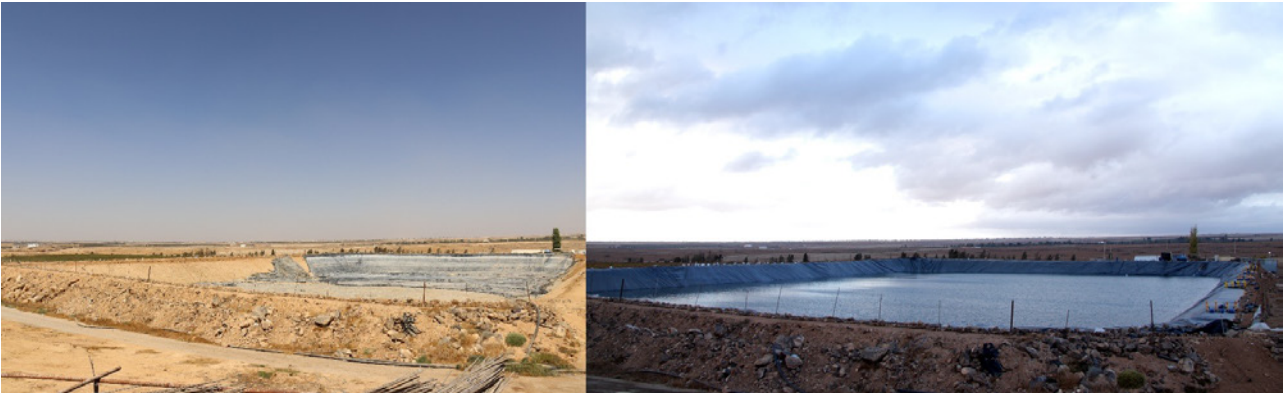
Figure 14: An agricultural water pond before (left) and after (right) rehabilitation
