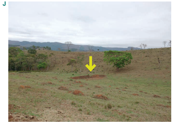
One of the 'small dams' built to slow down the outflow of the rainwater and to enhance soil water retention.
