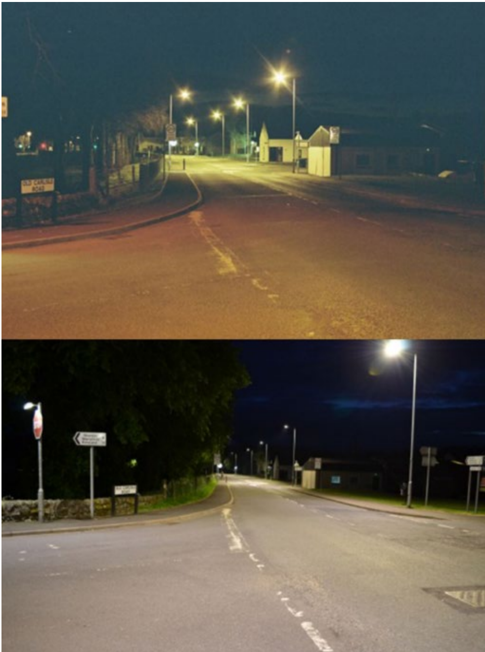
Figure 3.17. Views from The Holm, Moffat, UK, before and after retrofit. Source: IDA
