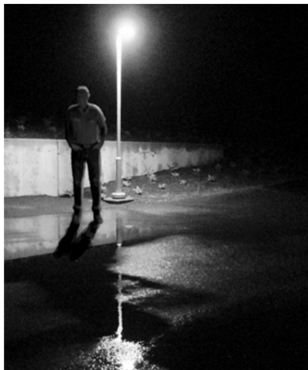
Figure A4.2. Poor shielding casts glare and creates pools of darkness. Source: Robert Dick
