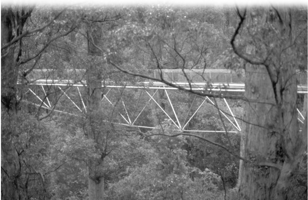
The elevated walkway in the Valley of the Giants in Walpole-Nornalup National Park in Western Australia was very carefully designed and constructed. The walkway allows park visitors to experience the upper reaches of a forest of giant tingle trees. Since construction of the Tree Top Walk in the national park, regional tourism has increased in the local area, and the environmental impact due to forest soil trampling has been reduced. Photo: Paul F. J. Eagles.
