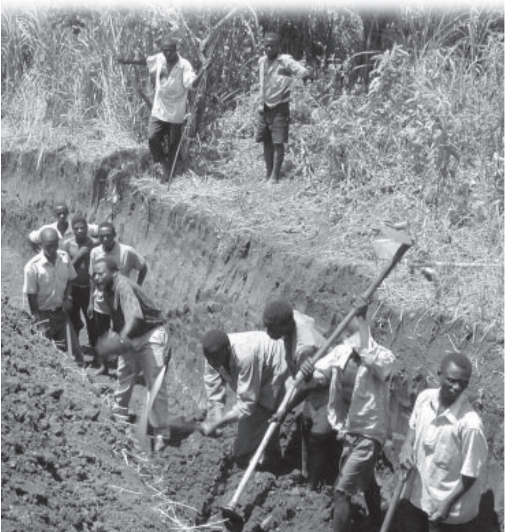
Building an elephant trench outside Kibale National Park. Photo: Purna Chhetri.
