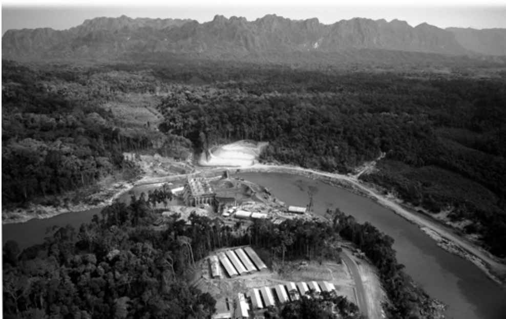
Theun Hinboun Dam, Laos, under construction. Photo: Stuart Chape.
