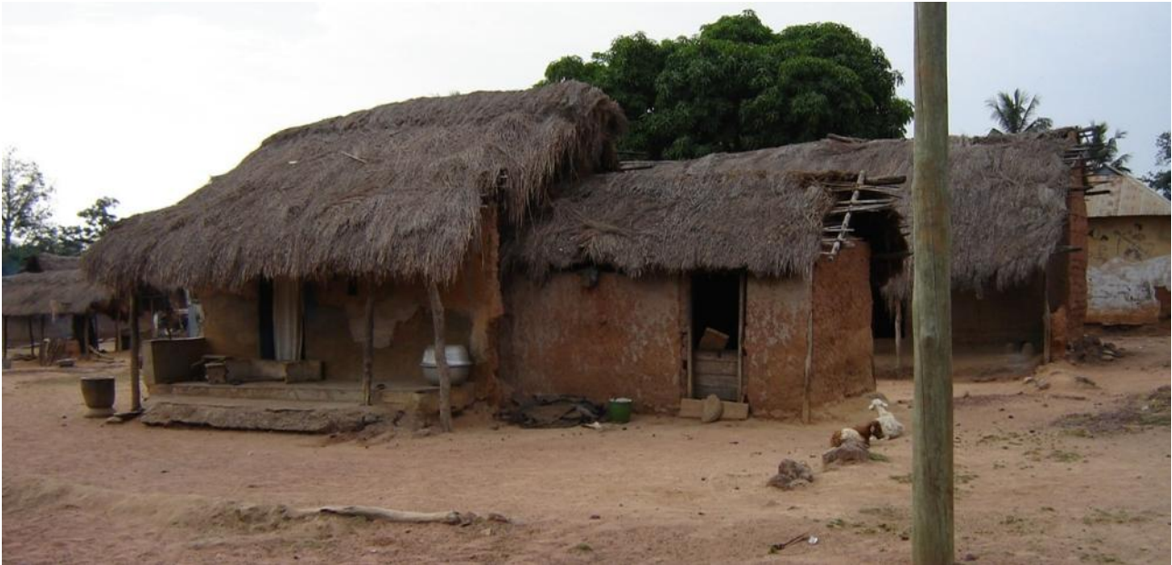
Mud/thatch houses are a common feature in the fringe communities of Digya National Park where poverty levels, according to national statistics, are relatively high © J. S. Ayivor
