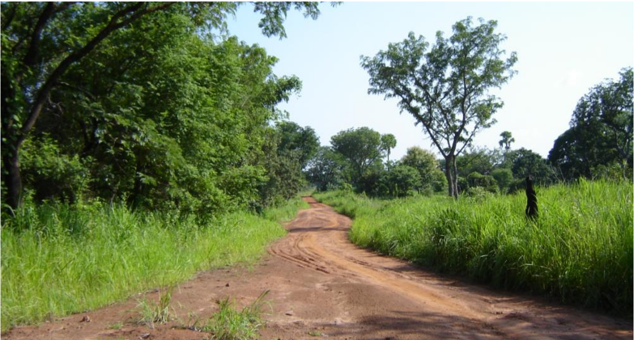
Access road constructed through the Kogyae Strict Nature Reserve for residents in the SUZ © Jesse Ayivor
