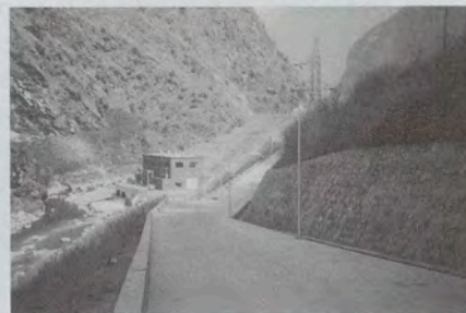
The Bhote Koshi Hydroelectric Project site
