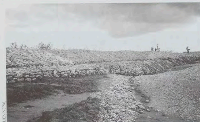
Spurs constructed along the rivulets in Ilam district have helped prevent crop damage during the monsoon
