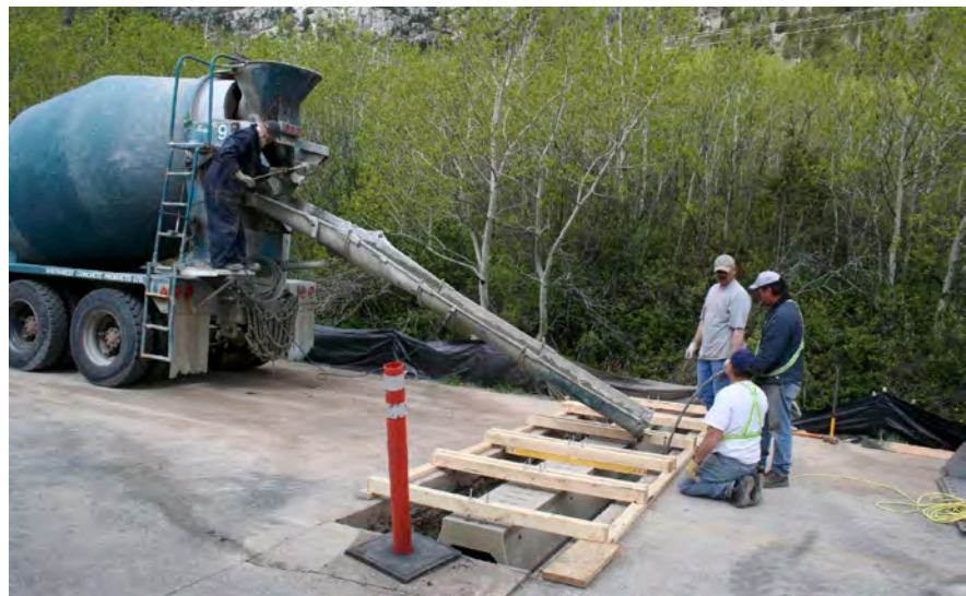
Construction of a salamander-friendly underpass tunnel in Waterton Lakes National Park, Alberta, Canada. © Cyndi Smith, Parks Canada
