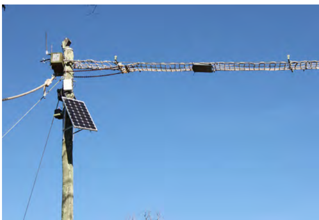
Wildlife cameras and passive integrated transponder (PIT) tags mounted at the end of a canopy bridge in Australia. PIT tag readers are technologies used to track the movement of individual animals that carry internal microchips. © Rodney van der Ree
