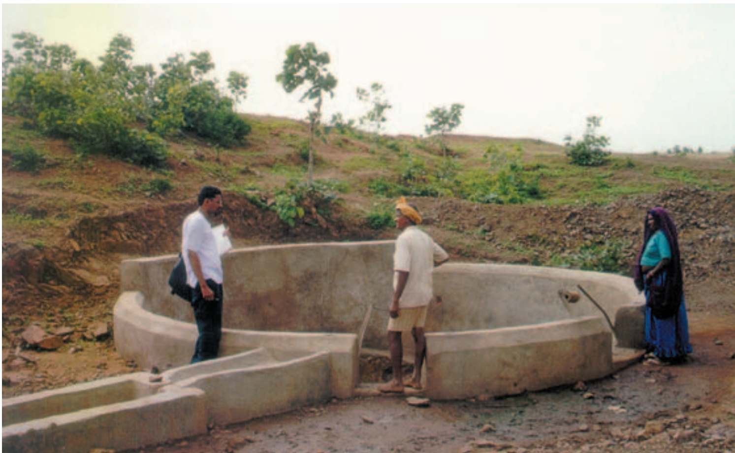
In dry climate tropics, agricultural yields may double by dryspell mitigation, based on supplementary irrigation, water harvesting and small-scale storage tanks.
