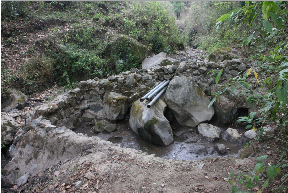
Fig. I-5. Creek bed below Bochojbo Alto, Chiapas. For most of the year a steady stream flows here, but during the winter dry season the flow stops. Locals have constructed a series of dams to hold water and pipe it away from the creek.
