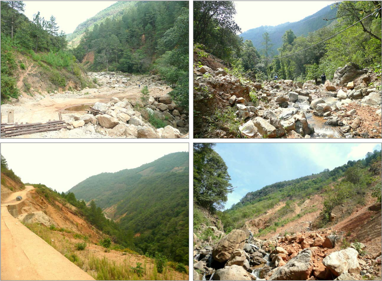
Fig. II-29. Río Alacrán (and an ill-defined construction site), where it meets the bend in the road 1 km E of Ayutla (top left). Flow along the Río Alacrán; note the large amounts of “new” rock material (top right). Road from Tierra Blanca to Ayutla above the Río Alacrán, showing its loose fill and evidence of landslides (bottom left). Looking upstream along the river at the type locality for Pseudoeurycea mystax ; note the overwhelming influence of landslides from the upper right (where the road cuts into the canyon wall) (bottom right).
