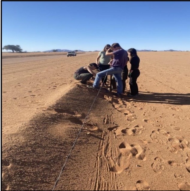
Figure 13: Installation of braided wire.
