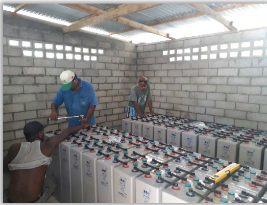
Figure 9: Batteries being torqued
