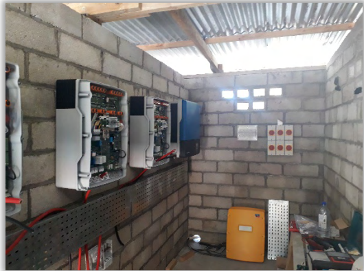
Figure 7: Inverters ready for wiring
