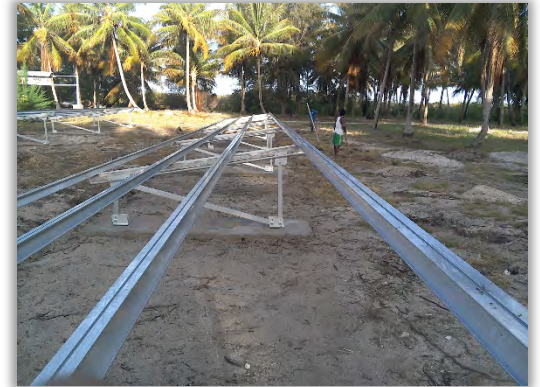
Figure 1: Mounting structure installed
