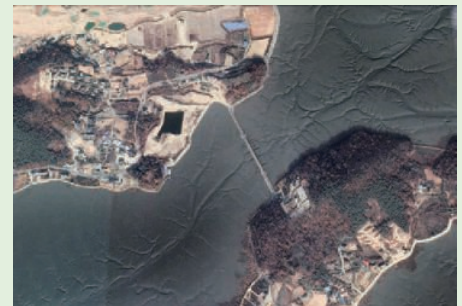
Current view of the bridge
