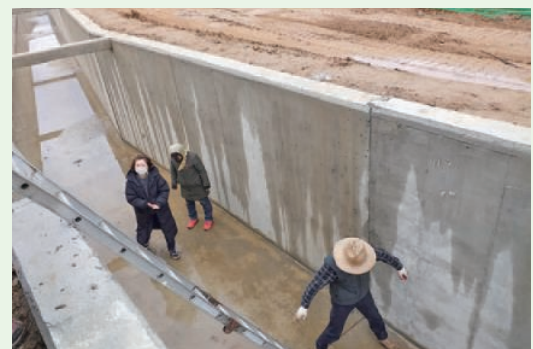
waterway made of concrete walls
