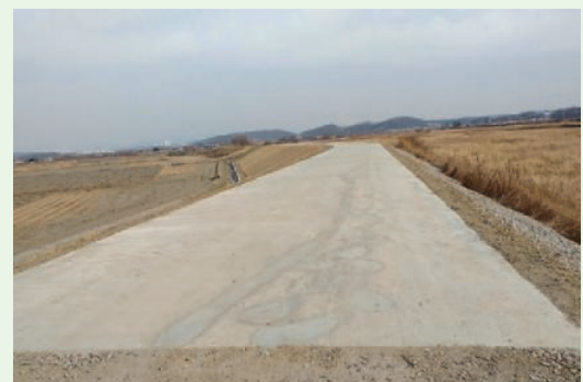
Embankment road widened to 7m
